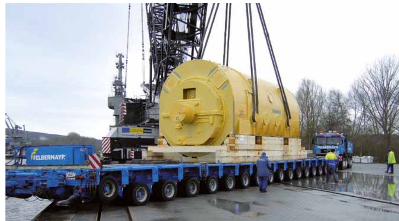
Loading of the components at the port Kehlheim
