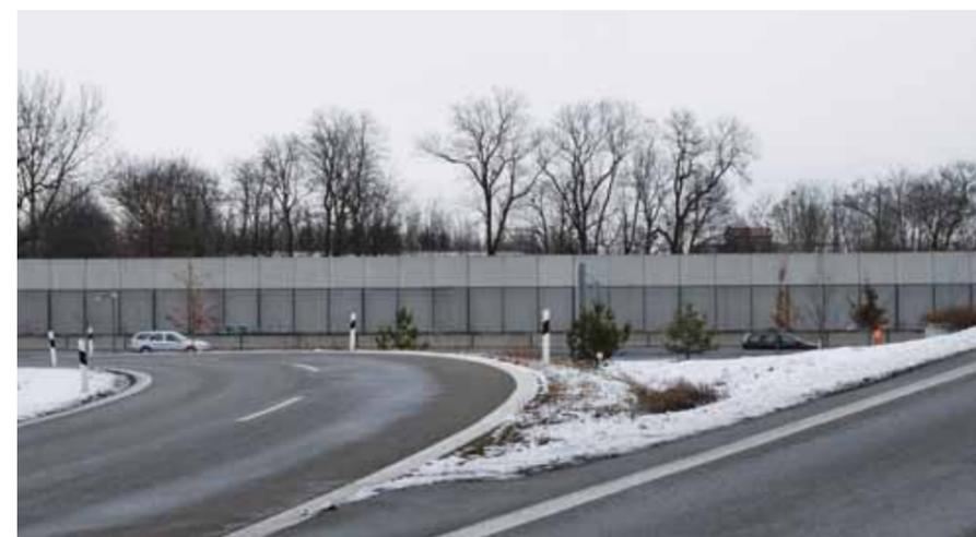
Concrete noise barrier with posts set in front – wire mesh screening – motorway A9 / Munich -Fröttmaning
