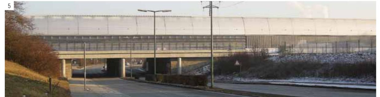
**1+2 Noise protection bridge with planar glazing fastened at individual points: motorway A9 / underpass Schleißeheim canal near Garching (Munich)**
