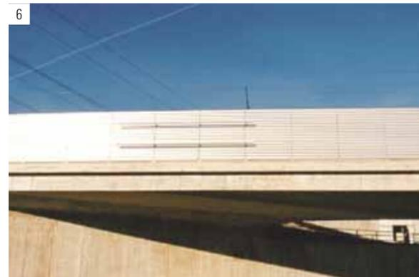
**1 Retaining wall with aluminium screening, embankment, concrete noise barrier with wooden battens and aluminium fitted to the side, height: 13 m; motorway A9 / Garching**
