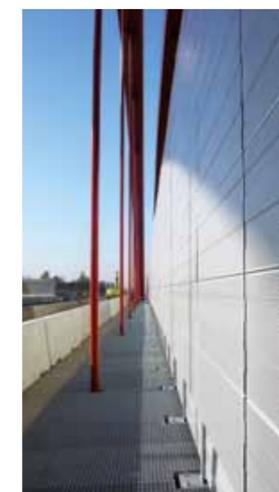
Aluminium cassettes with screening over the posts: motorway A8 west / middle barrier on the bridge over the Lech in Augsburg
