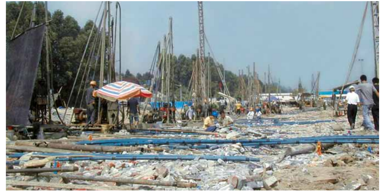
9 High-pressure injections near vertical shaft 1
