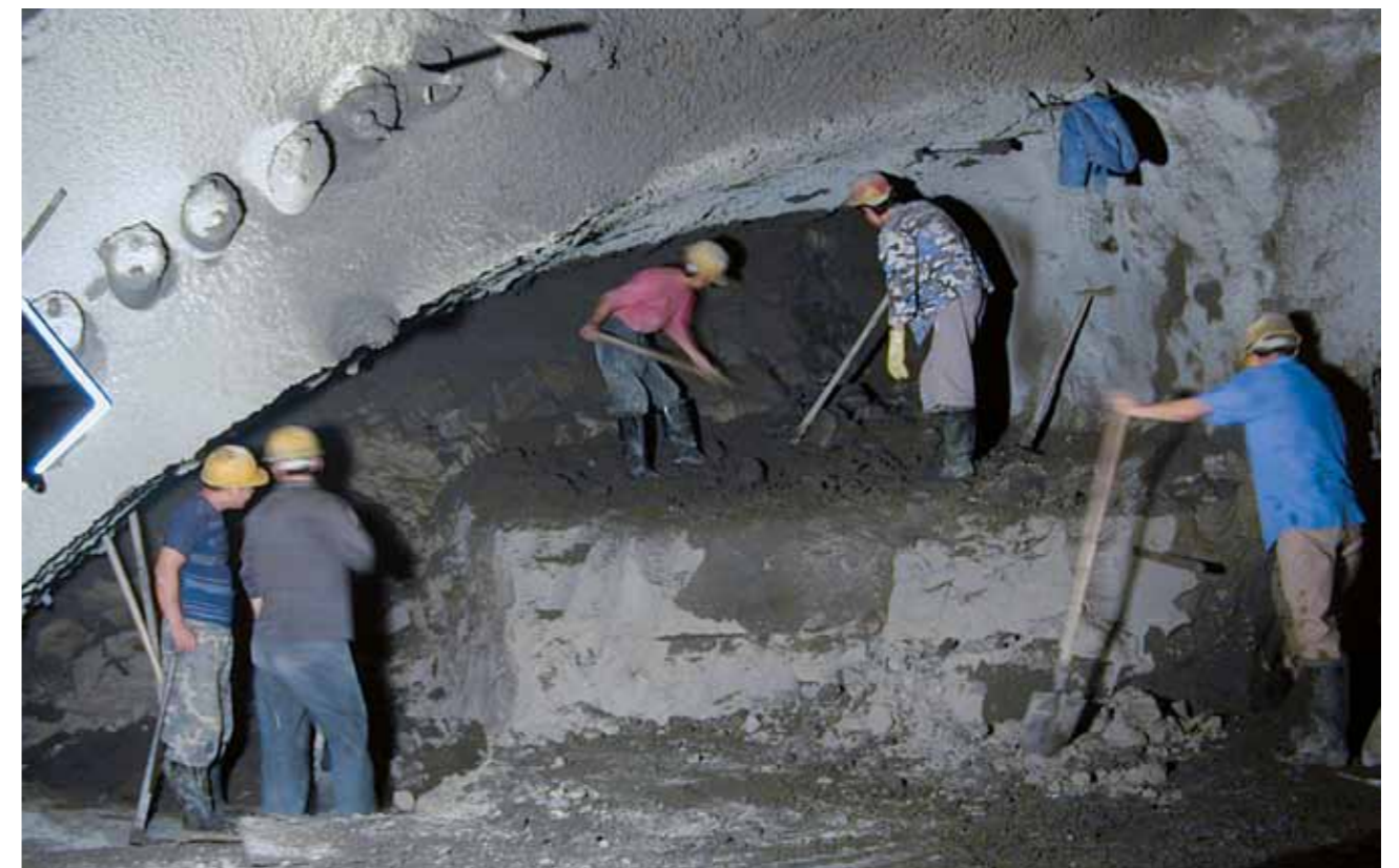
12 Mining by manpower in temporary shaft 3
