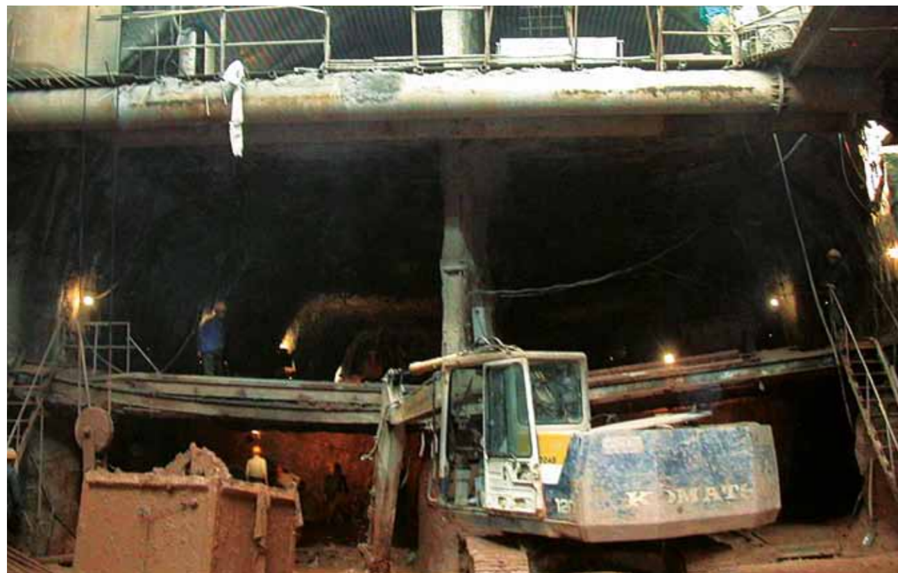
11 CRD method temporary shaft 3
