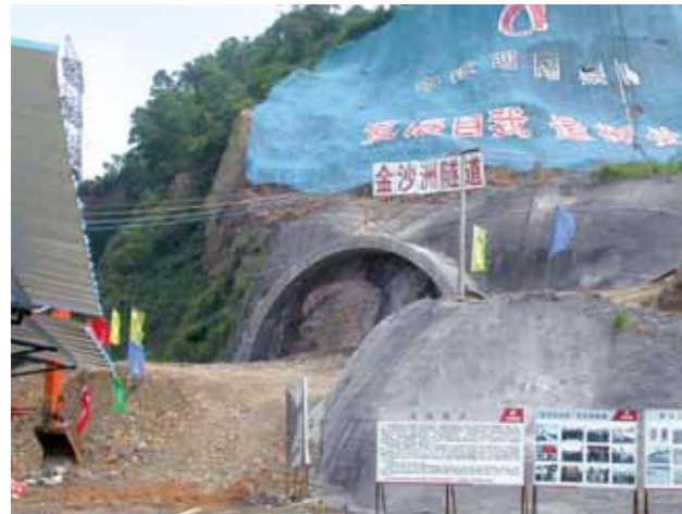
6 North entrance Jinsha Zhou Tunnel, beginning of construction 2006
